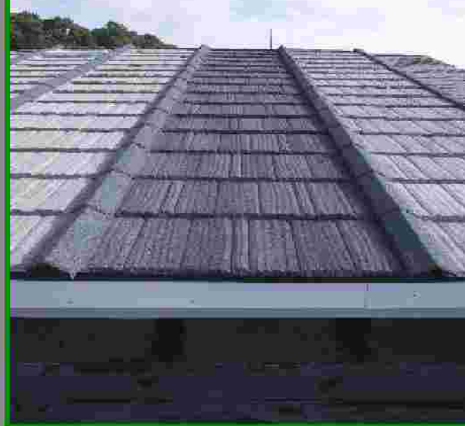
Dark Gray Shake, (SR08E90) Underside Unpainted Batten & Counter batten
